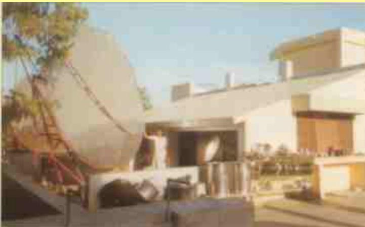
Barli has been successfully experimenting with solar cookers for over 15 years. Since 1998 the Institute has developed its kitchen tailored to solar cooking, and has installed 2 large Scheffler parabolic cookers in this kitchen. For about 300 days a year,
